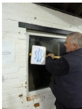
Dave using a suitable 'tool' to replace the window beading after temporary repairs.
