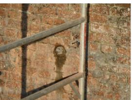
These two core samples were taken from the towpath side wall of Lock 14 for engineers to study the construction of the wall and the buttresses that support it.
