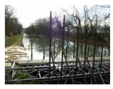
Photo (left) shows part of the 'Coffer Dam' mentioned last month. This type consists of a tubular metal frame which rests on both banks and a huge plastic sheet which is laid against it. The sheet, yellow in the picture (right), also covers the bank on each side of the canal. There are uprights to keep the whole structure in place but as can be seen, something that is relatively simple easily retains the half mile pound.
