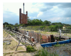
New gates are lifted in whilst we pump out the lock chamber
