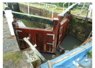
Balance beams are re-fitted. Final trimming up of gates
