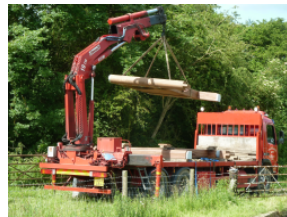
Lifting and moving the stop planks. Thanks to John Moulsher
