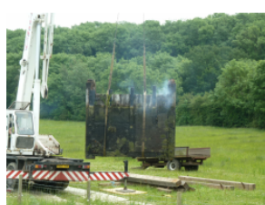
Removing the balance beam followed by the old gate, smoking from use of a grinder to cut away ironwork.
