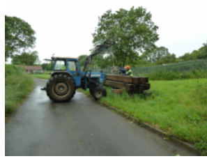
Lifting and moving the stop planks. Thanks to John Moulsher
