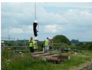
Removing the balance beam followed by the old gate, smoking from use of a grinder to cut away ironwork.
