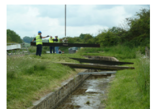
Lifting out the top stop planks for inspection
