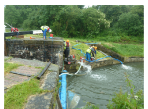
New gates are lifted in whilst we pump out the lock chamber
