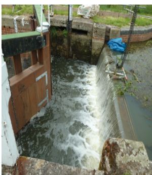
Final removal of top stop planks
