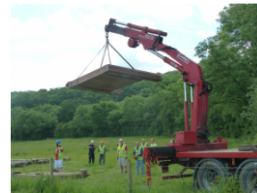
Lifting and moving the stop planks. Thanks to John Moulsher
