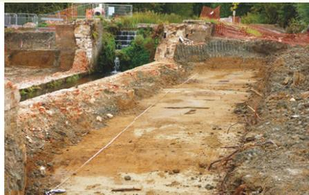
A lock with no walls! The next stage will be to excavate the footings for the new walls.
