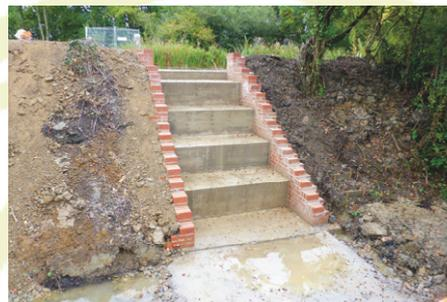
The by-wash, which is stepped to reduce the force of flow, when nearly completed.
