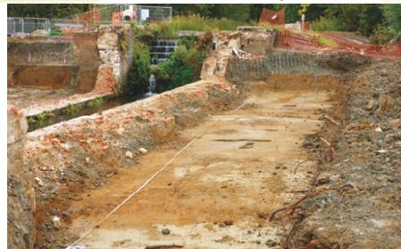
A lock with no walls! The next stage will be to excavate the footings for the new walls.
