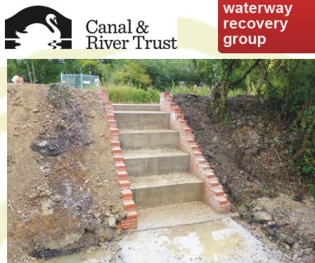
The by-wash, which is stepped to reduce the force of flow, when nearly completed.
