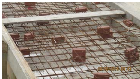
The reinforcement
