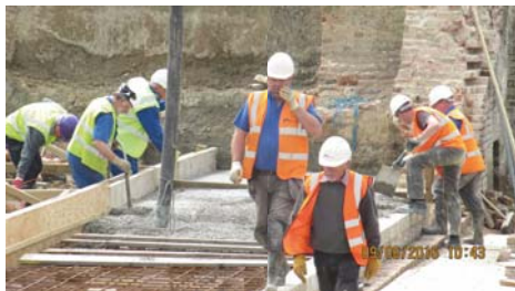
Pouring concrete - heavy work!
