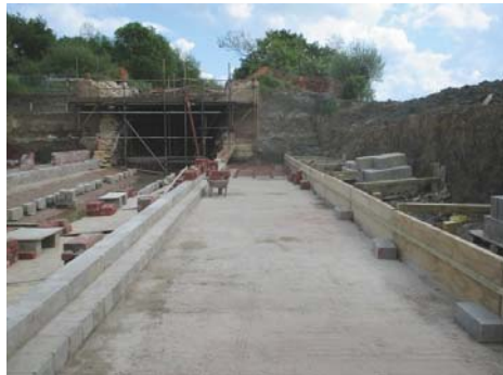
The offside ready for reinforcing steels
