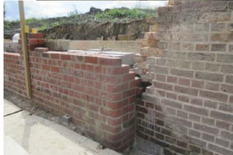
The gate recess is coming along nicely.
