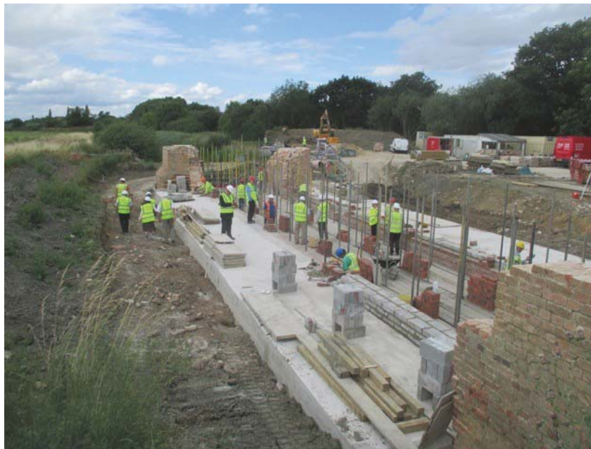
CRT executives visit site - and marvel at the progress!
