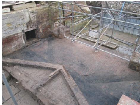
What a difference a weir (or removal of it) makes! After a difficult time breaking the very hard concrete the weir at Lock 15 has finally been removed – revealing beneath it an intact fore-bay floor in very good condition. The paddle-holes are also in good shape so not too much work required there either.
