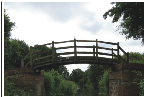
Casthorpe Bridle Bridge (c/o D Davis)
