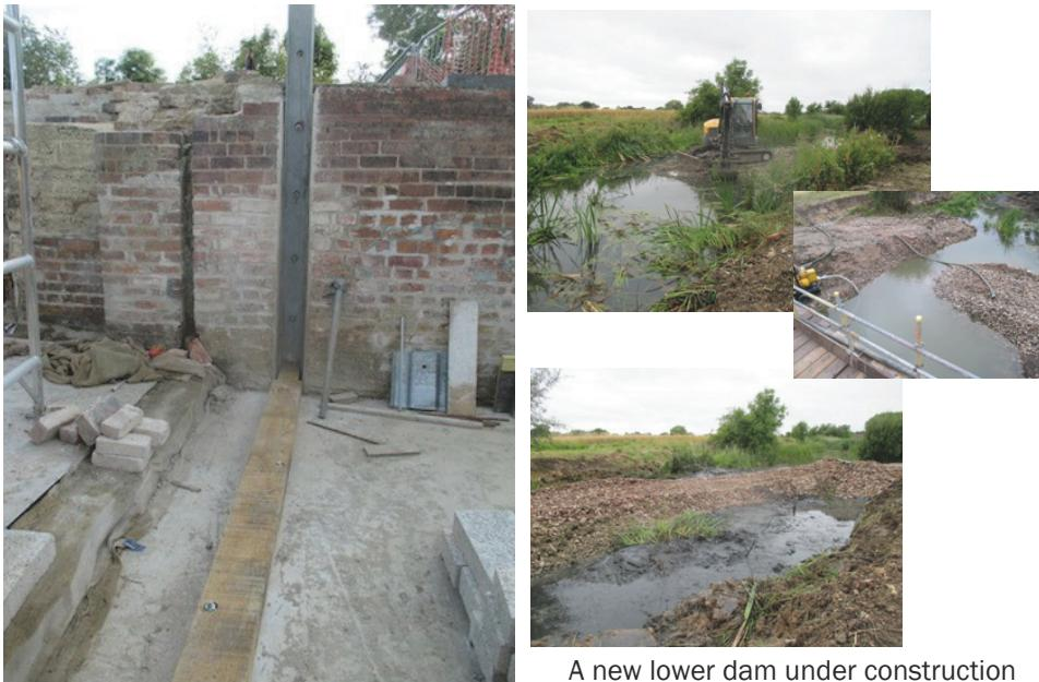
Stop board channels in place together with oak base timber.
