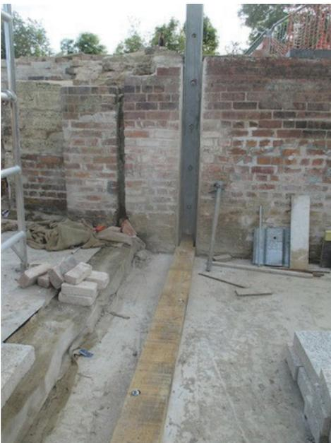
Stop board channels in place together with oak base timber.
