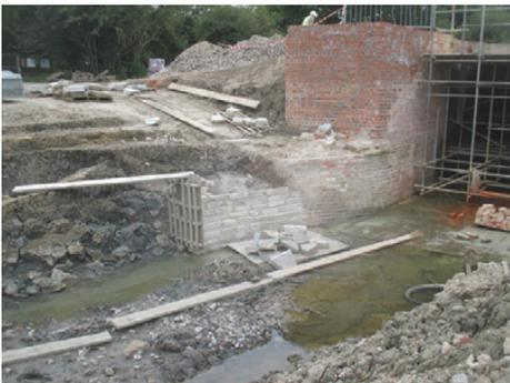
Lower near-side wing wall under repair
