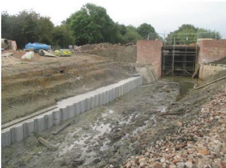
The foundations for the lock landing awaiting for the stonework to be laid.
