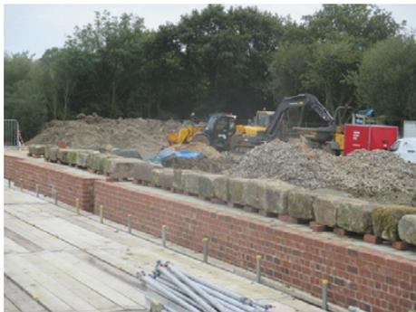
Coping stones being prepared on the off-side wall
