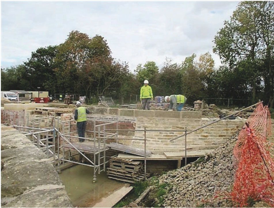
The GCS volunteer work party have just installed coping stones on the upper nearside approach wall.
