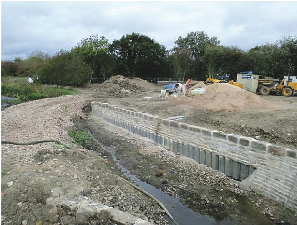
The completed lower mooring wall. Just some back filling needed then all that's required are the mooring bollards and the towpath reinstated.
