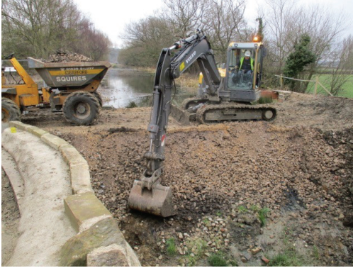
The clay lining is first removed
