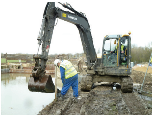
Tony and Rod setting the final level of the sheet piles that will form the edge the upper landing stage of lock 15.
