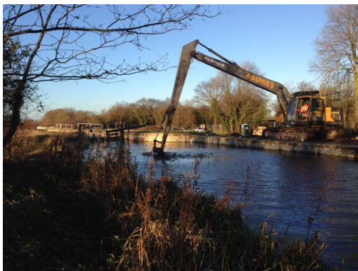
Dredging the pound between Carpenter's Lock & Woolsthorpe Middle Lock
