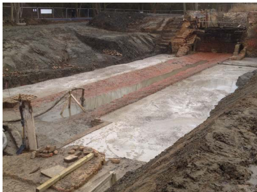
After the first concrete pour some tidying up and the whole area is ready for rebuilding to commence
