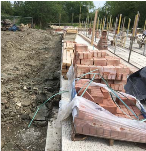
Nearly complete back filling showing the stepped concrete level after each pour
