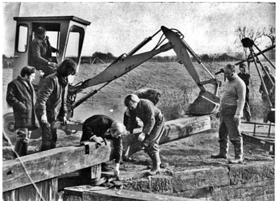
Refitting the old gates with help of the Smalley excavator
