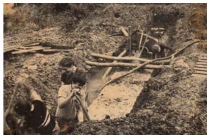
The test trench checking for leaks
