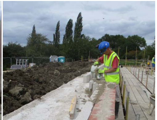
Philip grouting between bricks & blocks
