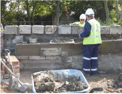
Richard and Rod adding coping stones to offside wing wall 17th Sept
