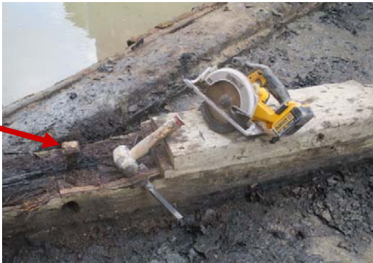
Removing the solid oak mitre beams which were held in place by 6 massive 18th C nails
