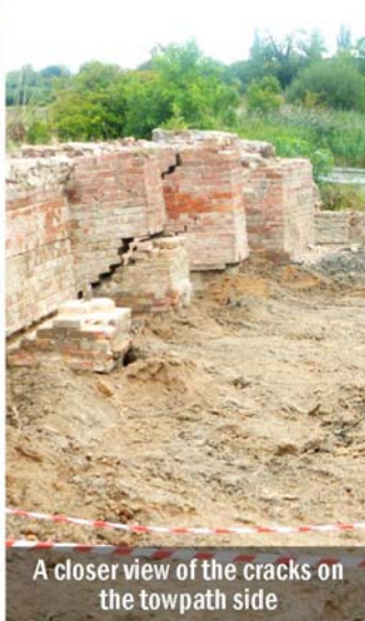
Buttresses exposed to reveal dangerous cracks
