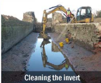
The invert finally exposed
