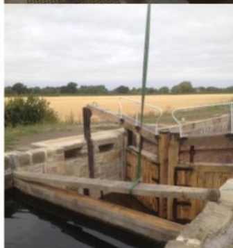
Stank planks being lifted before the lock is flooded August 2018
