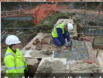
Dave & Iona work on the base of the nearside upper quoin
