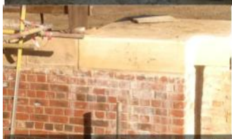
Anchor blocks fitted Sept 2017
