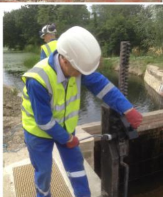
Checking the paddle gear
