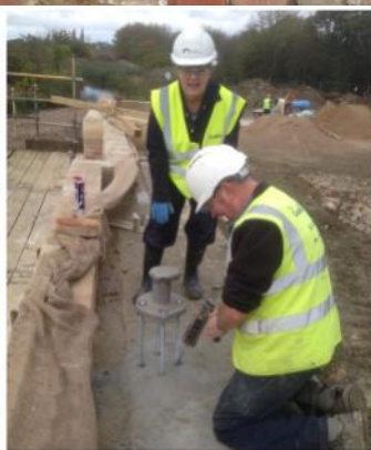
Mooring bollards being fitted
