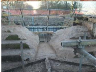
The weir gets demolished
