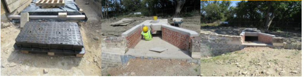
The byewash nears completion with just inspection covers now to be fitted
