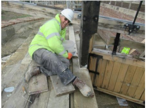
John grouting around the paddle mechanism
