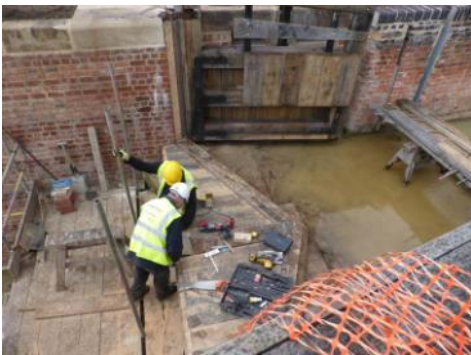
Rod & Keith fitting the mitre boards
