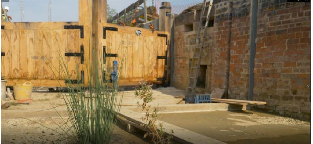
Some screen shots from the video of the top gates being fitted at Lock 14. Filmed by Sea Lane Media Ltd (Aerial photos & video) www.sealanemedia.co.uk
