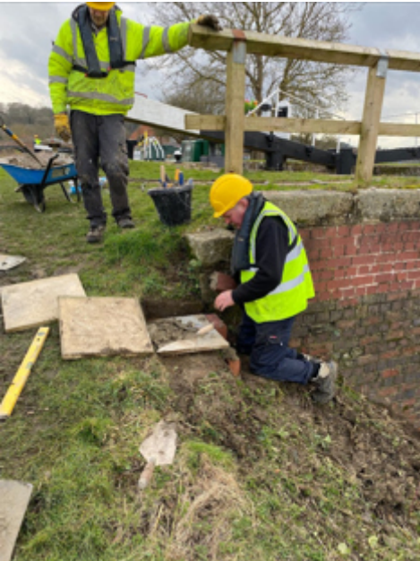
Lock 16 towpath side to put in the new steps – Lou completing 2nd step (Feb).
