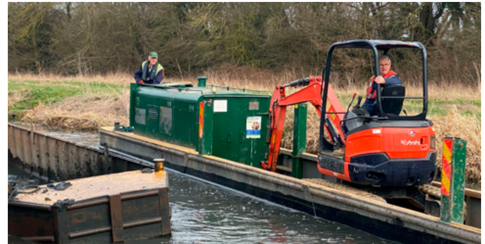
Betty with the on-board excavator during silt removal works.
